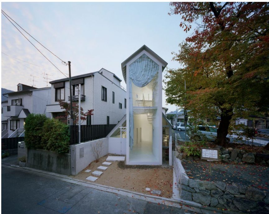
Figure 1. Installation view of Curtain for O House (2009). The large curtain for the façade covers a window of W2 × H7.1m, this to ensure the privacy of the residents and also insulate the window further against cold air. ©Takumi Ota
